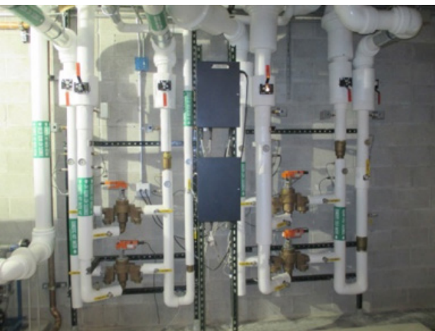
Acorn BASyC system that features two SFMMV supply fixtures, installed at Northwestern Medicines - Lake Forest Hospital
